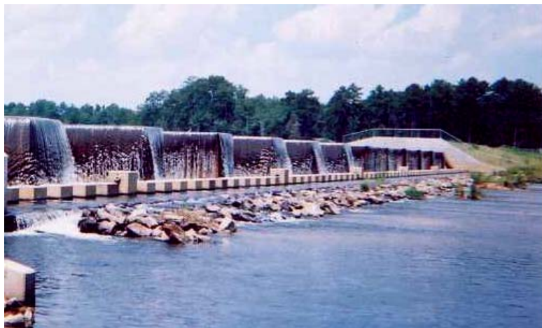
Fig. 7 - Full height labyrinth, Whitewater Lake Dam
