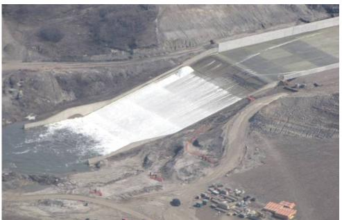
Figure 5: 2009 Spring Flood Passage Through Partially Replaced Spillway (Phase I / Existing)
