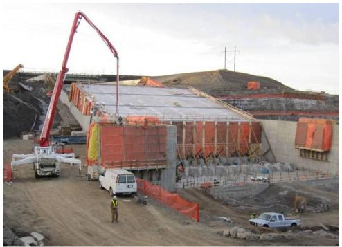
Figure 7: Hoarding for completion of Phase 2 Spillway Concrete and Anchoring in 2010
