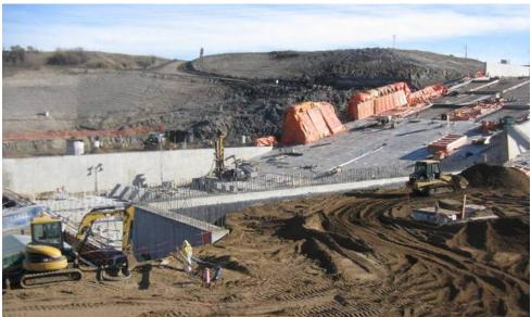
Figure 6: Phase 2 Spillway Chute and Basin Construction Underway in 2009
