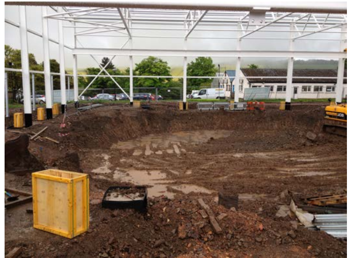
Fig. 5. Initial excavation of pit for the containment tank with the steel frame of the building erected before excavation commenced.
