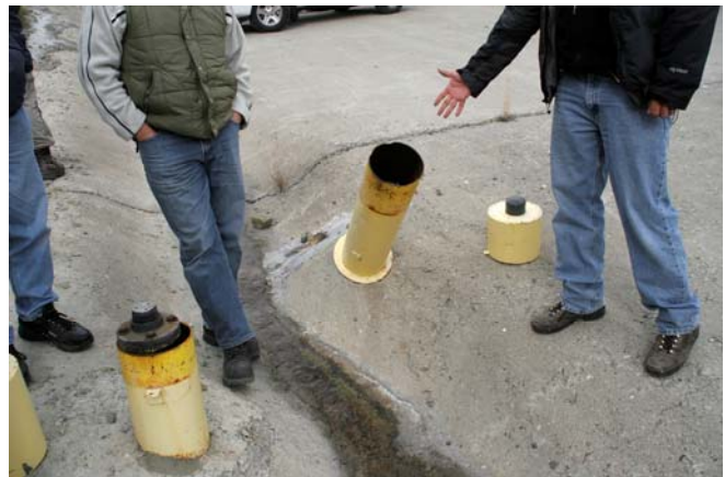
Photo 8: Vertical extensometer (on left, showing head) and inclined extensometer (in middle).
