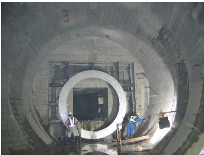
Figure 4: Headrace Access Tunnel Opening
