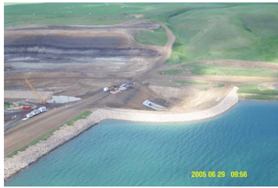
Photo 8: South Dam Outlet Structure with Upstream Cofferdam
