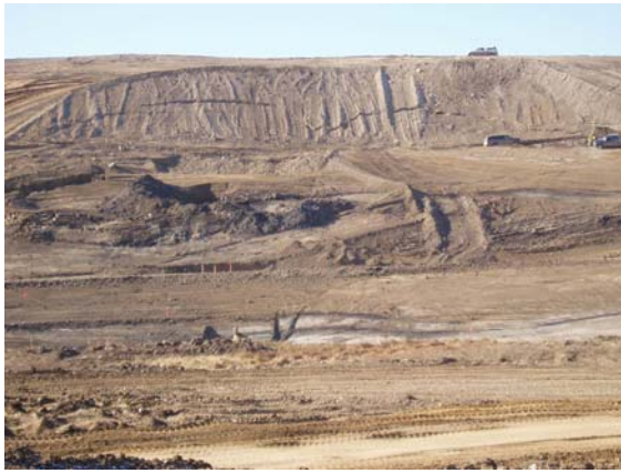
Photo 7: McGregor South Dam West Abutment Slide Scarp
