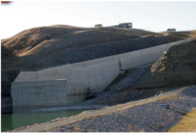
Photo 3: End of spillway and flip bucket.
