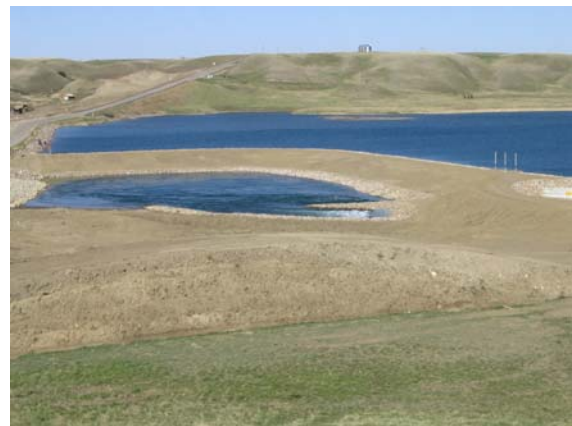
Photo 4: Lomond Crossing Cofferdam and Control Structures in Operation
