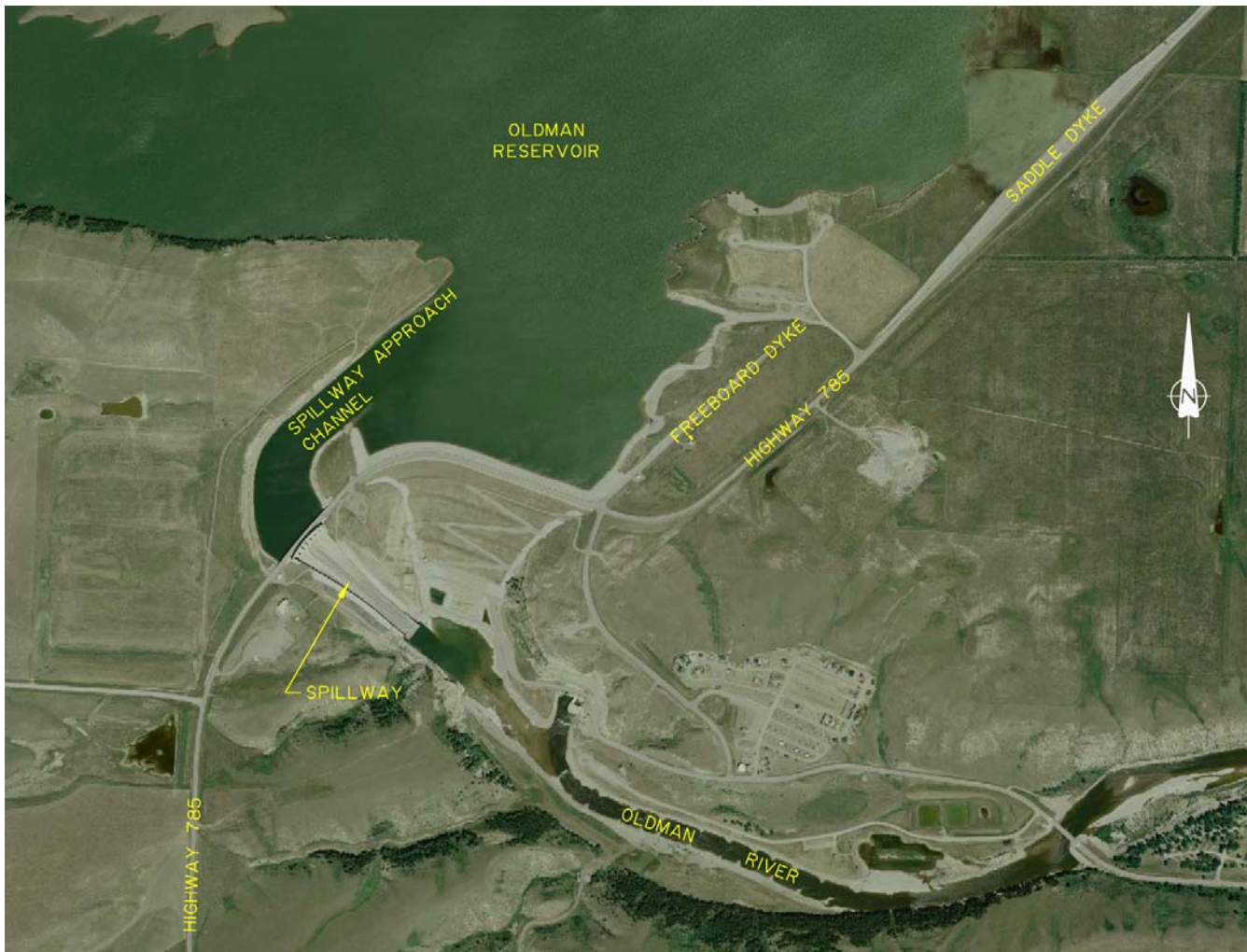
Figure 2: Layout of Oldman Dam and Spillway (Photo courtesy of Tarin Resource Services Ltd.)
