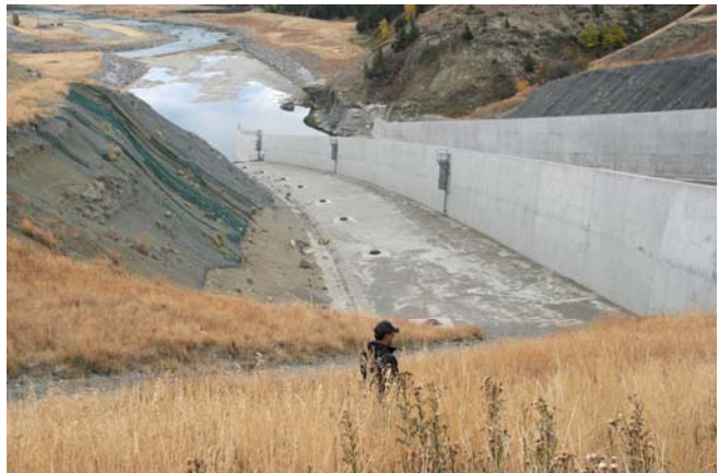
Photo 6: Left side of spillway, showing manholes for drain
