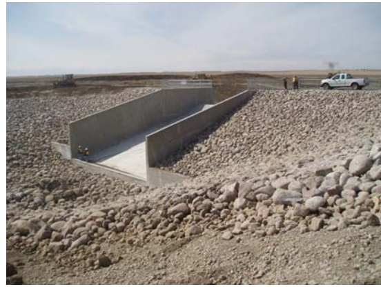
Photo 2: Completed Drop No. 4 Structure
