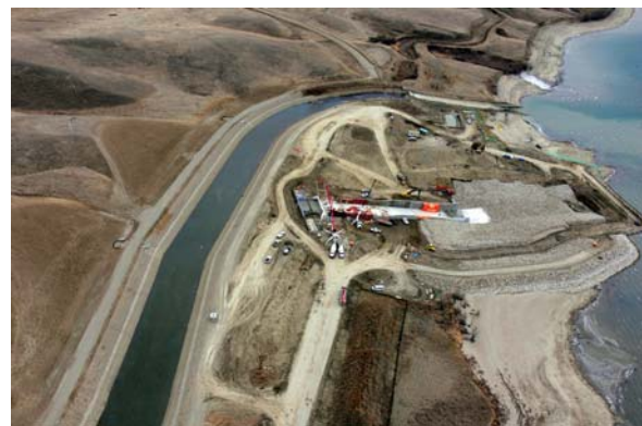
Photo 12: Travers Inlet Structure Partially Completed
