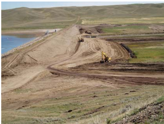
Photo 5: McGregor South Dam Stripping
