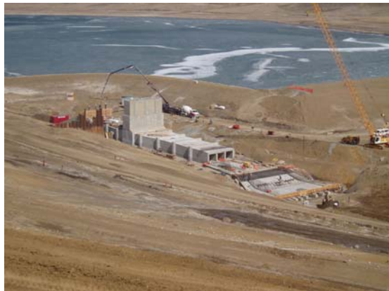
Photo 9: McGregor South Dam Outlet Structure
