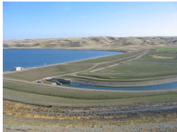
Photo 10: Completed South Dam and Outlet Structure
