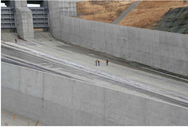
Photo 1: Spillway walls and floor.
