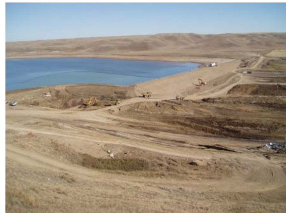
Photo 6: McGregor South Dam Outlet Structure Excavation.
