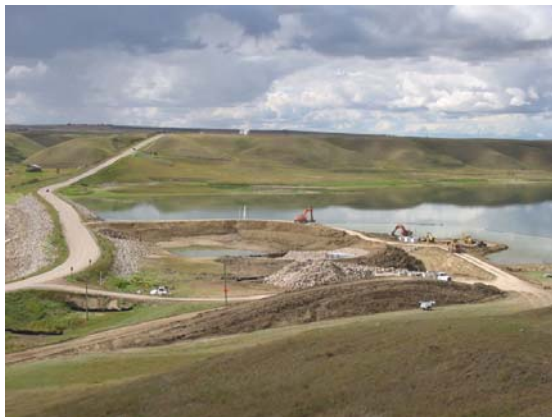
Photo 3: Lomond Crossing Cofferdam Under Construction
