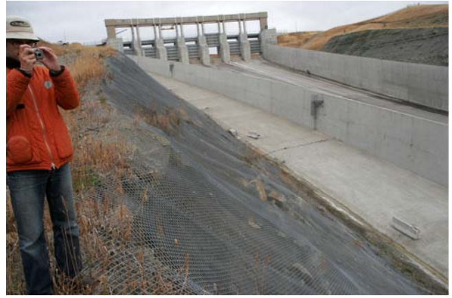
Photo 2: Right side of spillway, showing mud slab, spillway walls and head works.
