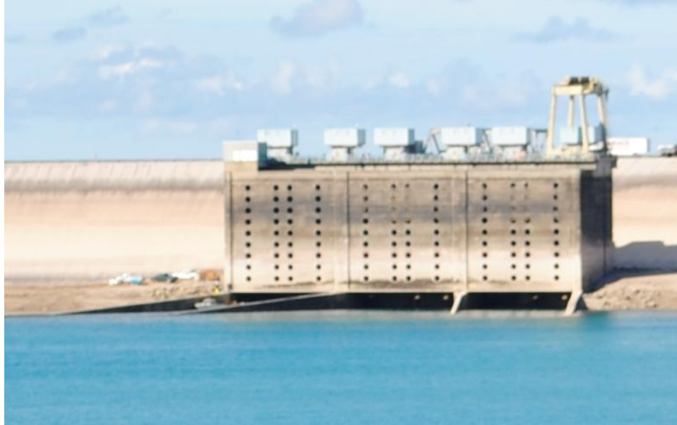
Figure 4 : Prototype Intake Structure
