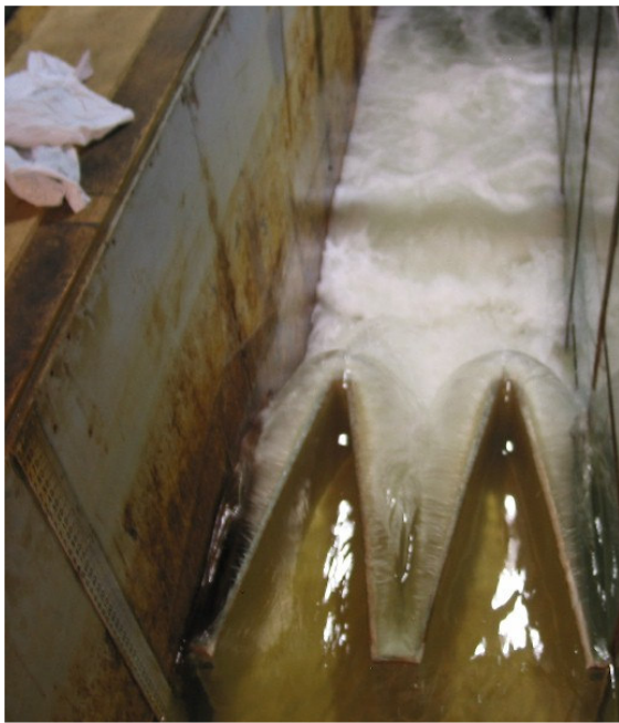
Figure 3. - View looking down on the 2 cycle labyrinth discharging 53,000 ft 3 /s over the embankment.
