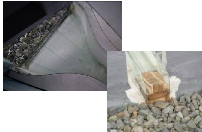
Figure 5: Images from above the flume entrance and flip bucket
