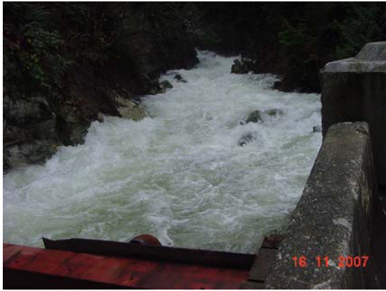
Figure 2: View looking upstream of the existing flume entrance
