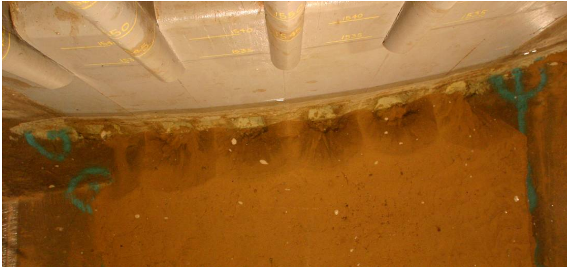
Fig. 9. Flushed area near bottom outlets after sudden gate opening.
