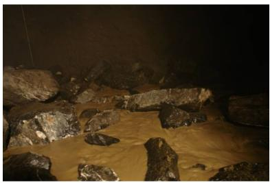
Figure 2: Water inrush in karst tunnel gushing
