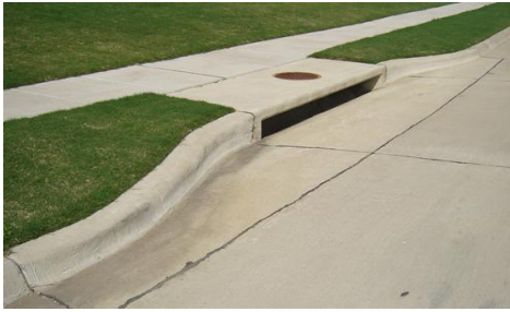
Figure 2.1 Example of Curb Inlet
