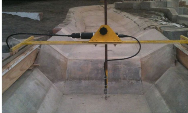
Figure 5. Trial Smooth Spillway
