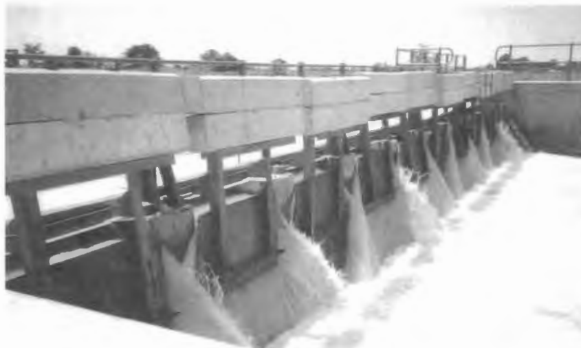
Figure 6. Ten Begemann gates in the Hadejia Valley Irrigation Project North Main Canal (Litrico et al., 2005)
