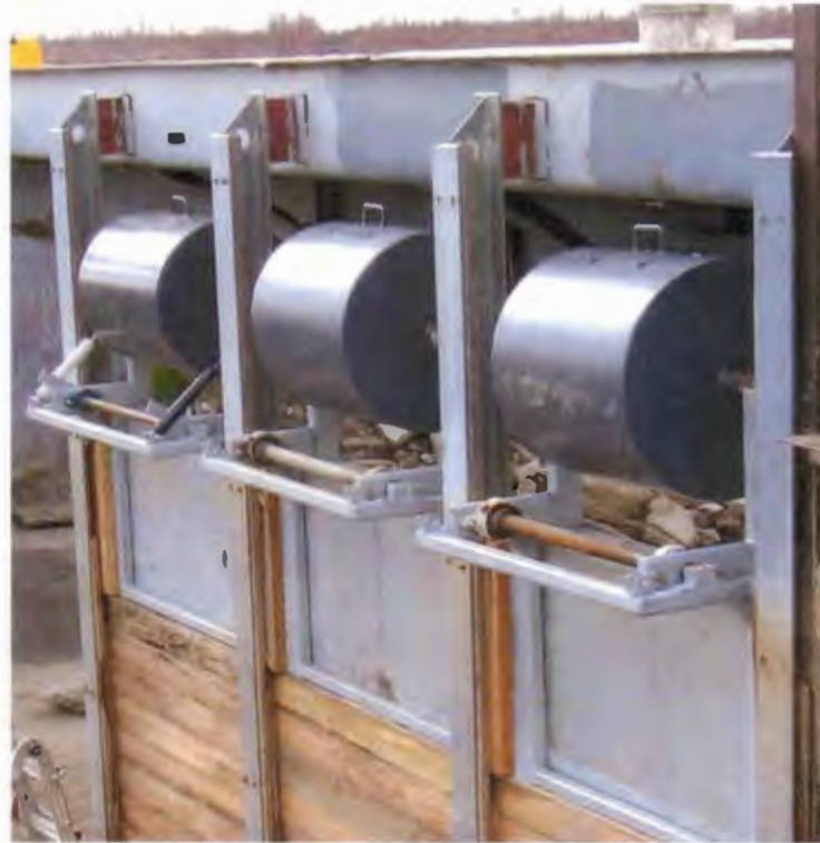
Figure 13. Installation of ITRC Flap Gate in a flashboard structure (ITRC, 2013)
